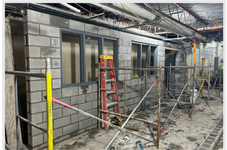
Findorff masonry crews, alongside MEP crews, working to build interior walls that will provide new spaces in the Test Kitchen/Head House areas.
